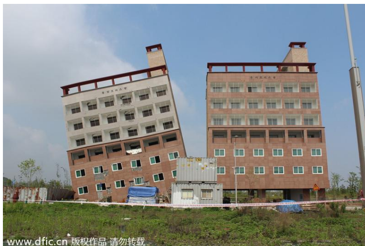
Slika 13. Urušavanje zgrade uslijed hidruličkog sloma tla ( http://www.chinadaily.com.cn/world/images/attachement/jpg/site1/20140513/0013729e42d214dbcd5116.jpg ). Datum pristupa: 24.5.2018
