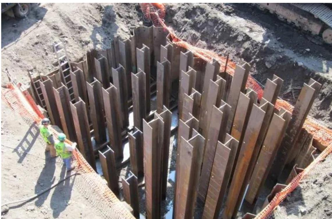
**Slika 10.** Čelični piloti (<https://theconstructor.org/structural-engg/foundation-design/steel-piles/40266/>)
