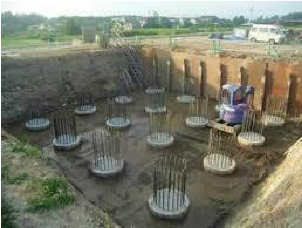
Slika 12. Armiranobetonski piloti ( https://www.structuralguide.com/concrete-piles/ )
