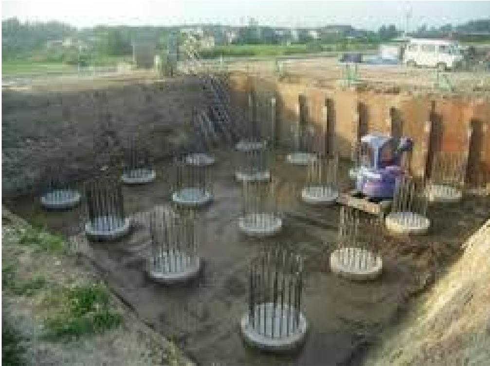
**Slika 12.** Armiranobetonski piloti (<https://www.structuralguide.com/concrete-piles/>)
