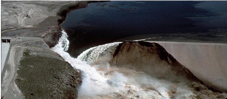
Slika 8. Slom brane Teton(Perrow,1984)
