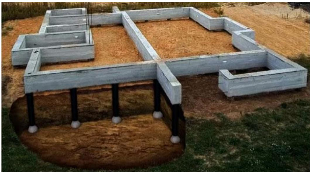
**Slika 8.** Drveni piloti (<https://hourstrong.com/pile-temelj-drvenih-pilota/>)
