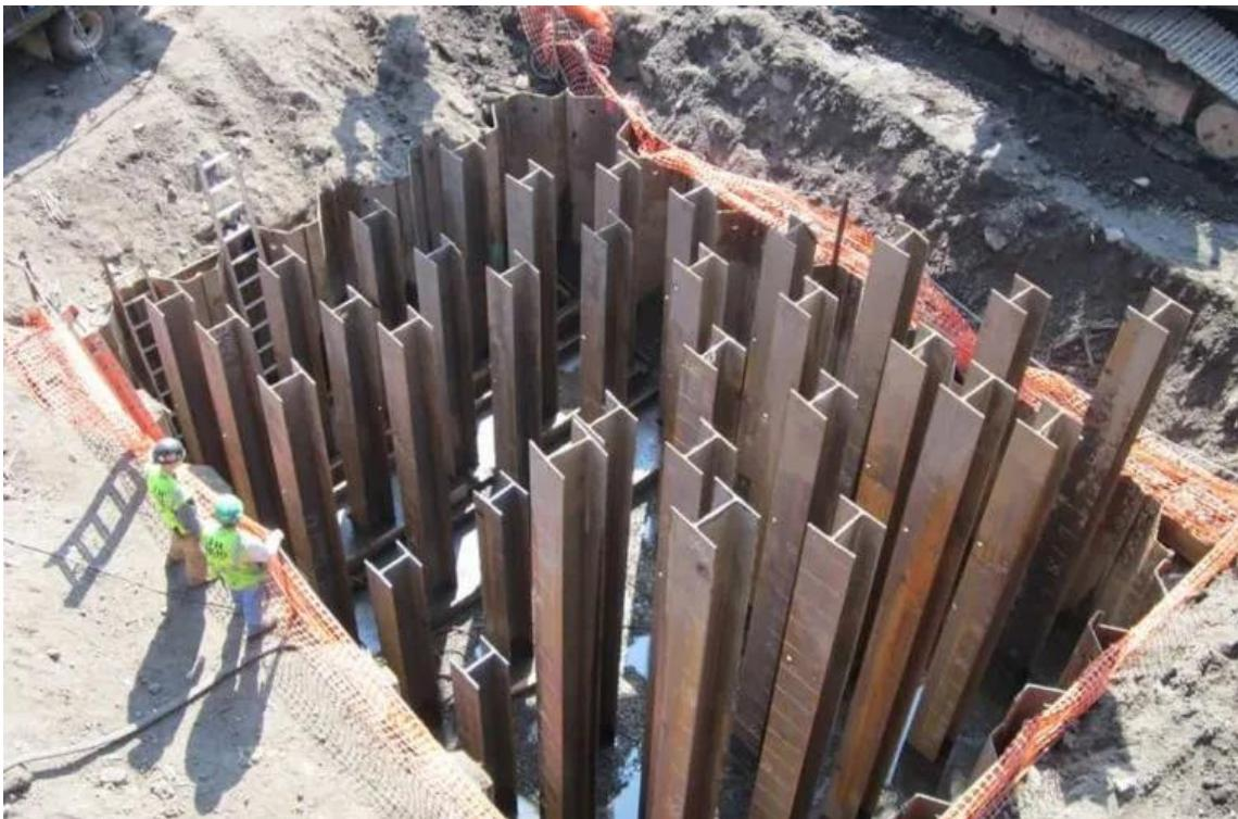
**Slika 10.** Čelični piloti (<https://theconstructor.org/structural-engg/foundation-design/steel-piles/40266/>)
