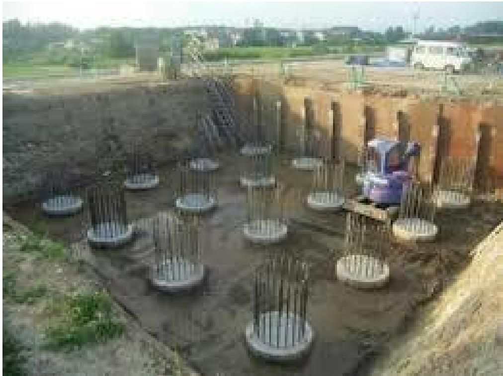
**Slika 12.** Armiranobetonski piloti (<https://www.structuralguide.com/concrete-piles/>)
