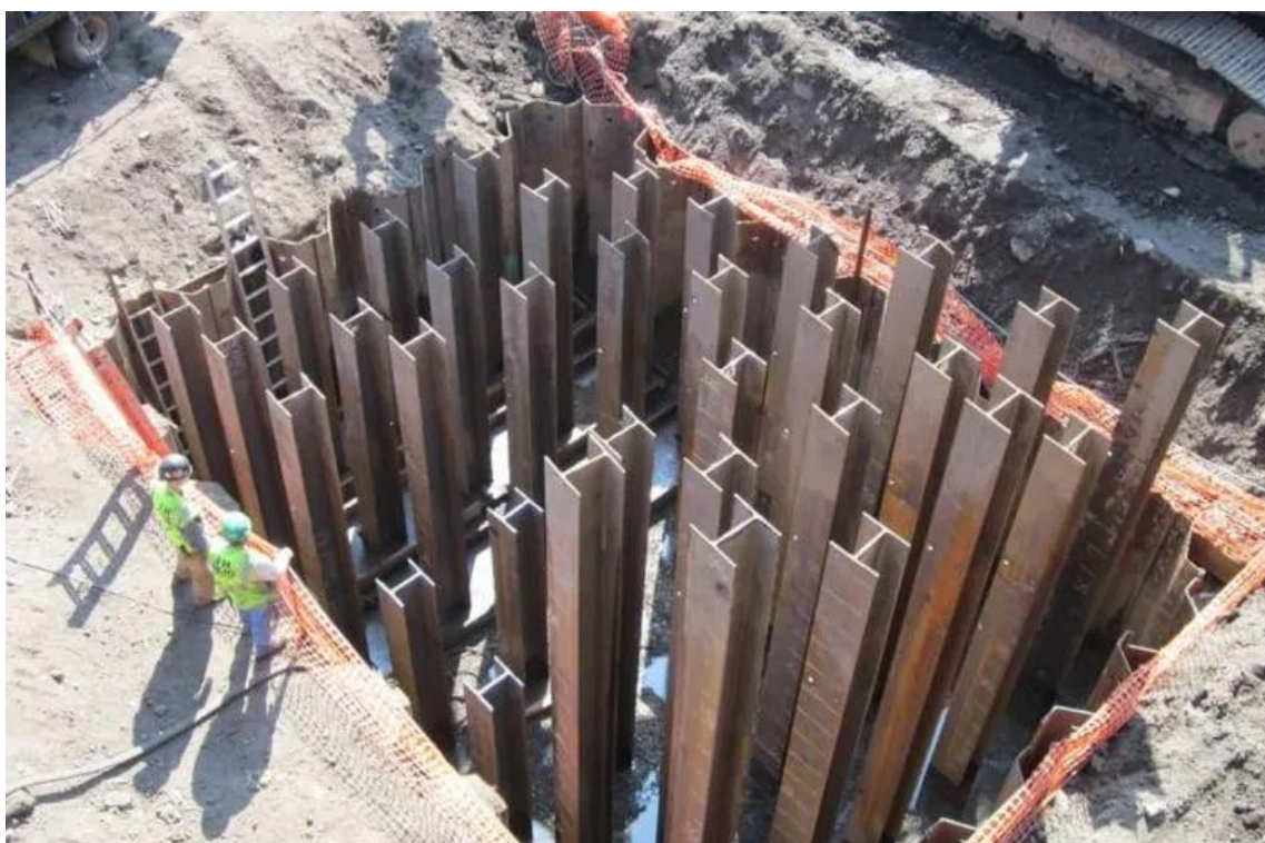
Slika 10. Čelični piloti ( https://theconstructor.org/structural-engg/foundation-design/steel-piles/40266/ )
